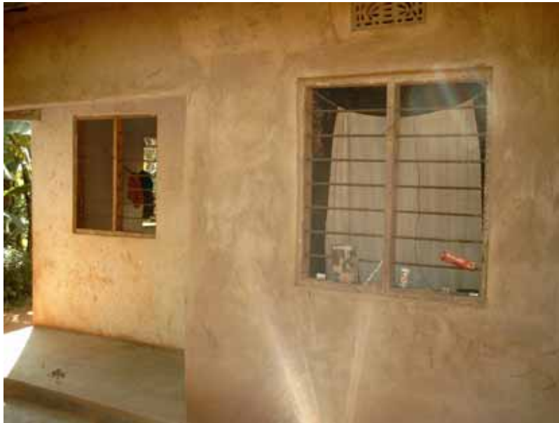
A house of a widow at Kirimeni who is living with four orphans constructed under Ha YaMwi building fund.
