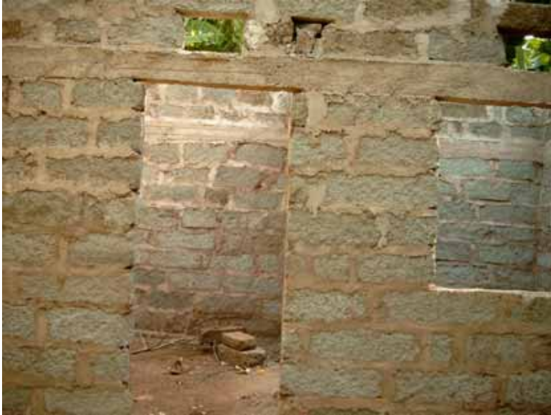
New house of a widow at Kirimani congregation on construction.
